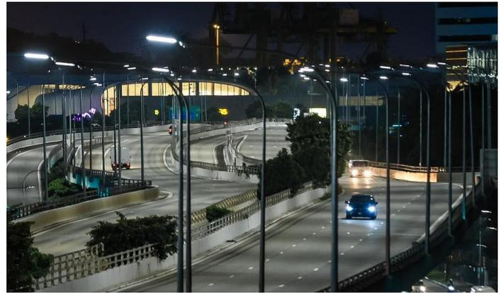
**APR – Sustainability.** As part of its green transport and energy conservation efforts, LTA completed a year-long effort to replace the orange glow of conventional street lamps with a more energy efficient lighting system using clear Light-Emitting Diodes (LEDs).
