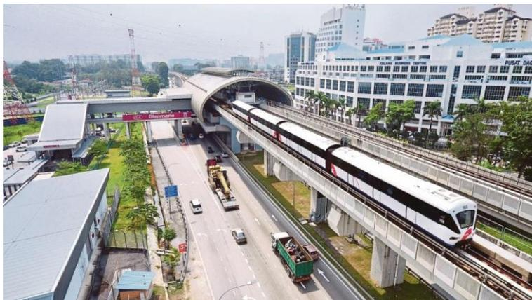
**FEB – Rapid Transit System (RTS) JB-SIN:** Progress continues to be made to complete the 4 km rail shuttle service, connecting Singapore and Johor Bahru by end-2026. The RTS has the capacity to carry up to 10,000 pax per hour in each direction and will be connected to Woodlands North MRT Station.
